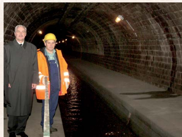
Lord Mayor Heinz Fenrich and an employee of the Stadtentwässerung (city's department for drainage) at the opening of the visitors' area of the Landgraben in Lameyplatz in 2002
