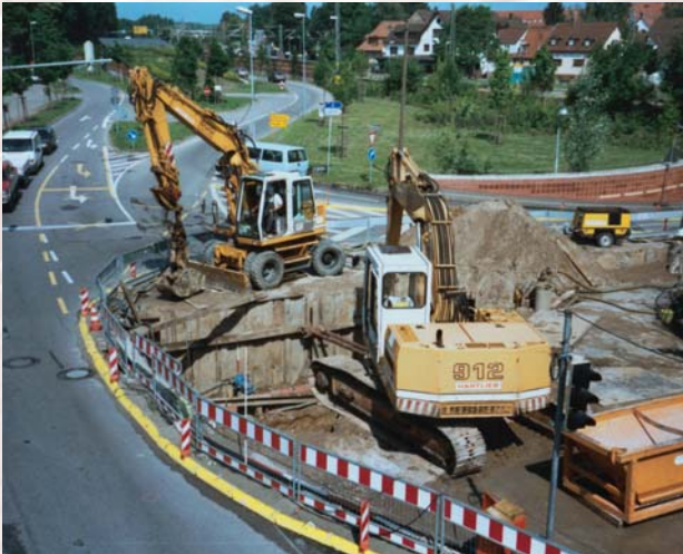
Traffic obstructions during using the cut-and-cover method
