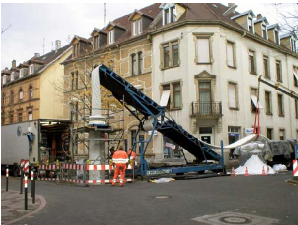
Inserting the plastic tubing
