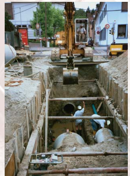
Pipe replacement using the cut-and-cover method
