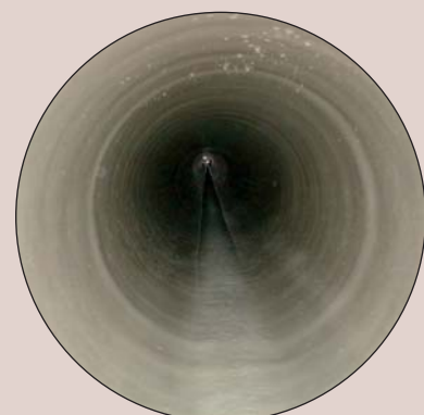
After renovation: a pipe lined with glassfibre-reinforced plastic
