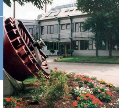
The wastewater treatment plant administrative building
