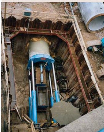
Thrust pit with hydraulic presses
