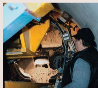
Excavating the soil at the site
