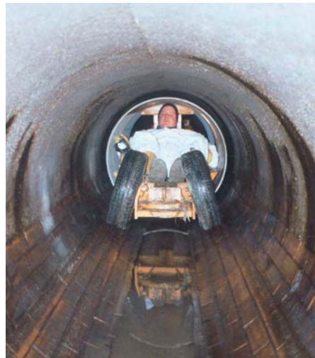
Inserting the pipe
