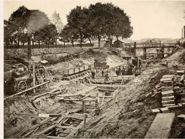
Steam powered pumps in operation during the "correction of the Landgraben"
