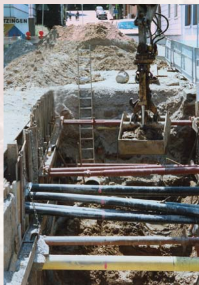
Supply lines complicate the work
