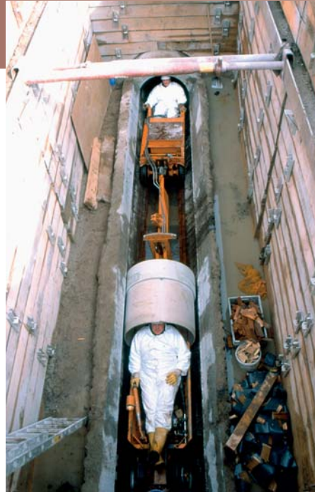
Insertion pit for pipe relining
